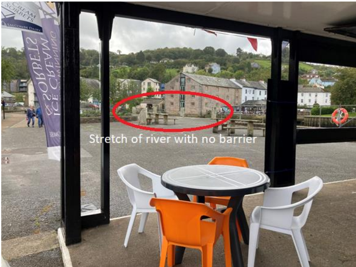
View from southern end of premises toward river
