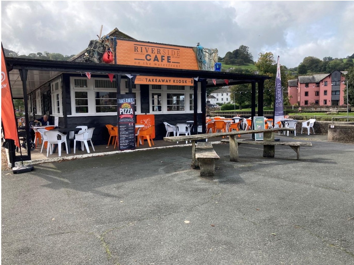
Northern end of premises
